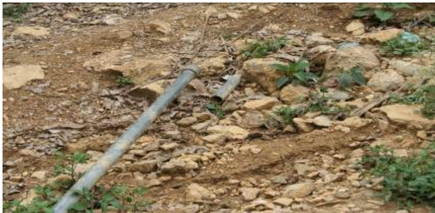
Figure 11: One of the broken water pipes for about 6 months in Hin Hon village, Pú Nhuồng resettlement site, Mường La district, Sơn La province
