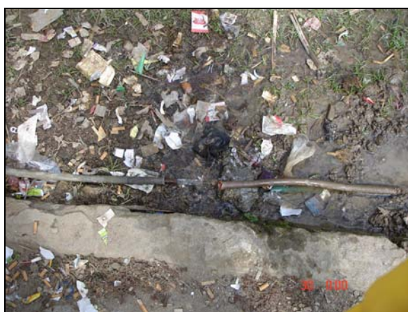
Picture 6: Water pipe from the mountain to household: it's broken and that makes the water contaminated.
