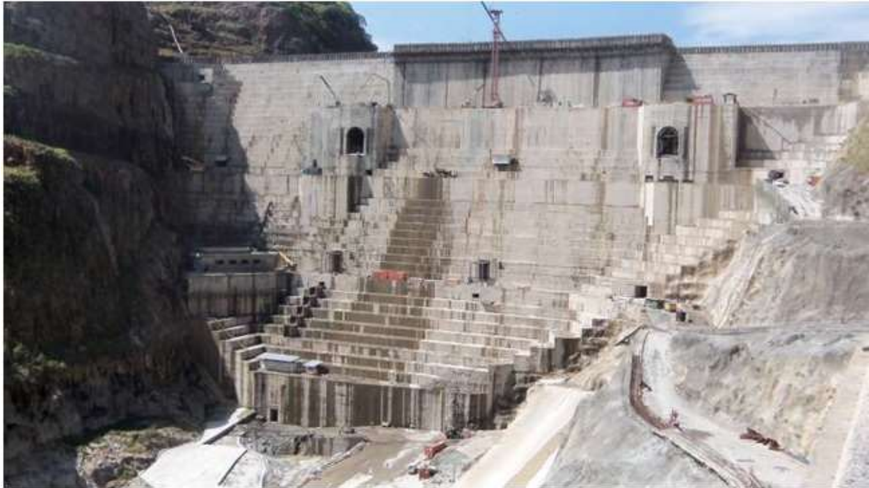
Figure 1: Gibe III dam under construction (EEPCo, 2012).
