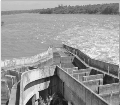
Failed fish pass structure at Pak Mun Dam, Thailand
