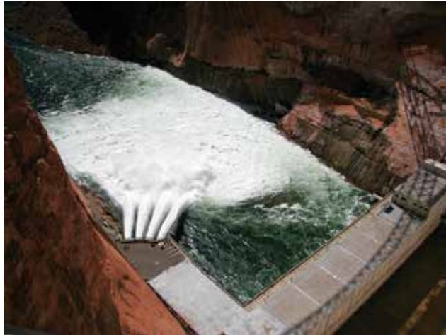
View from top of dam of all four jet tubes open releasing water for high-flow experiment - March 5, 2008
